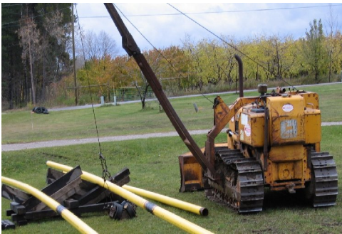
Natural gas pipeline project
